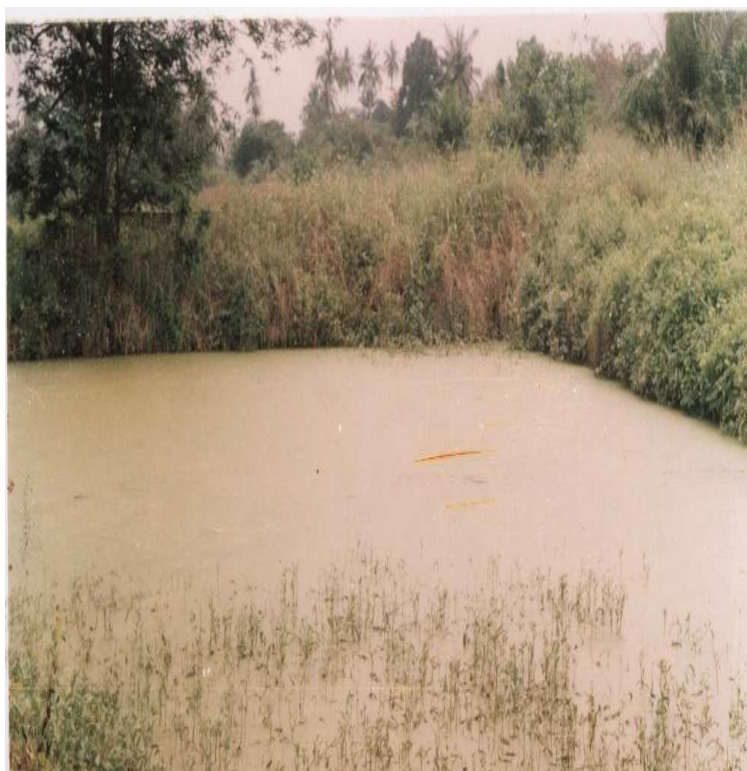
Figure 2: Slide showing part of the Leachate Lagoon.
