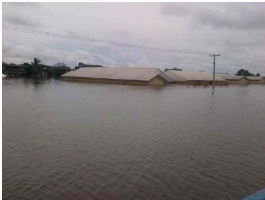
Plate 1.2: Picture of area with total submergence by flood [10].
