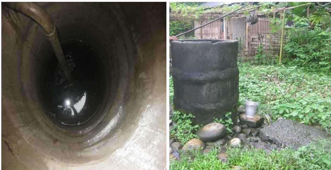
Figure 1. Drinking water sources in the affected areas (Wells without brim or platform)
