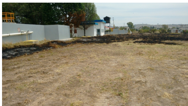
Figure 1: Area destined for the treatment of the static cell in situ .
