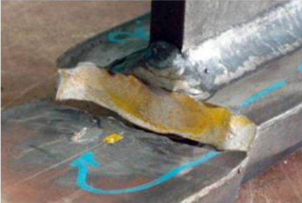
Figure 1: Example of steel fatigue failure.
