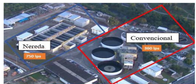
Figure 3: Comparison of flow capacity versus area between Nereda and conventional.
